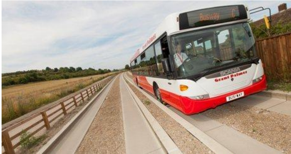
Figure 6: Luton-Dunstable Busway (courtesy of Luton Borough Council)
