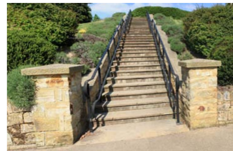
Steps / stairs from central events space
